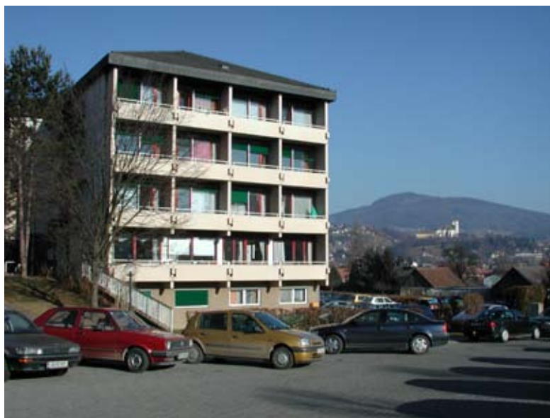
Fig.1: Old People's Home before and after its renovation
