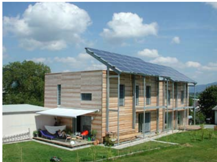
Zero Energy Houses in Weiz
