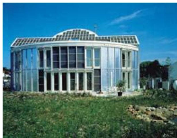
Figure 2: The Energy Autonomous House, Freiburg 1991
