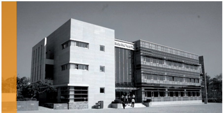
A Korean green building (Kolon E&C Institute of Technology) including geothermal heat pump, building integrated photovoltaics, double-skin, light shelves, solar tubes and natural ventilation, etc.
