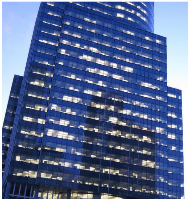
Figure 1-1: A large office building façade, showing the juxtaposition of the occupant-controlled window shades and the operator-controlled lighting
