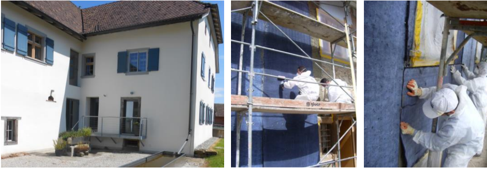
Figure 3-4: Old mill renovated in Oberhallau, Switzerland [54].
