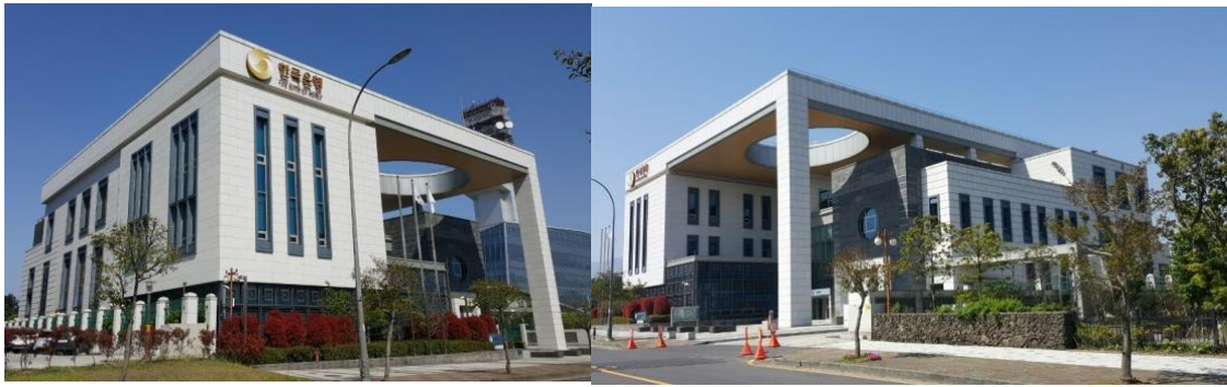
Figure 3-22: Jeju branch of Bank of Korea. (Photo: Jun-Tae Kim).
