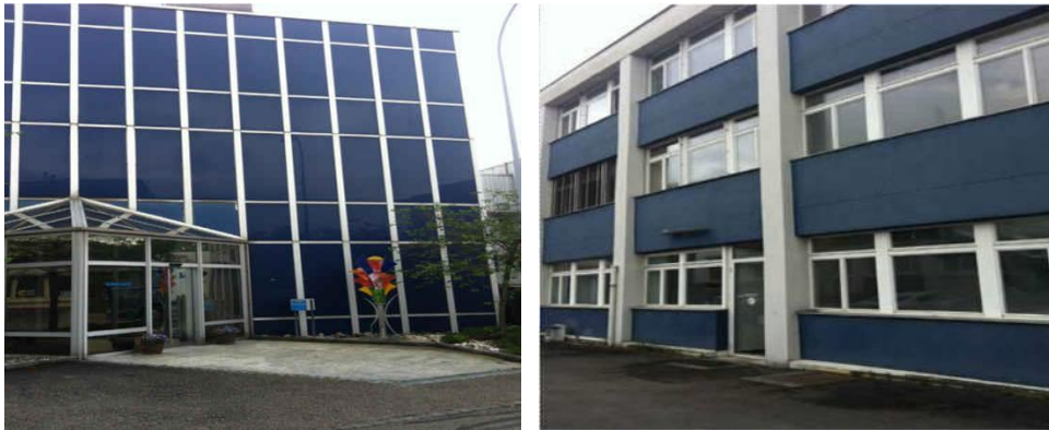
Figure 3-9: Office and production site in Switzerland [59].
