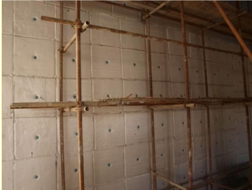
Figure 3-12: Wuxi video city with VIPs in the walls (Photo: Zhaofeng Chen).
