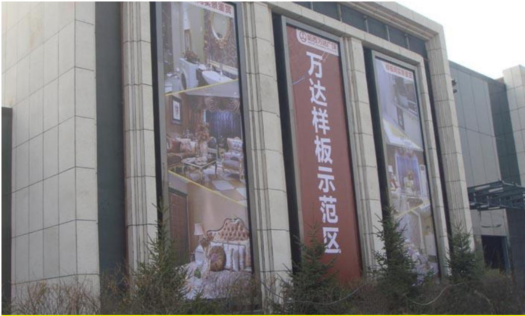
Figure 3-10: Wanda plaza where walls and roof were equipped with VIPs (Photo: Zhaofeng Chen).
