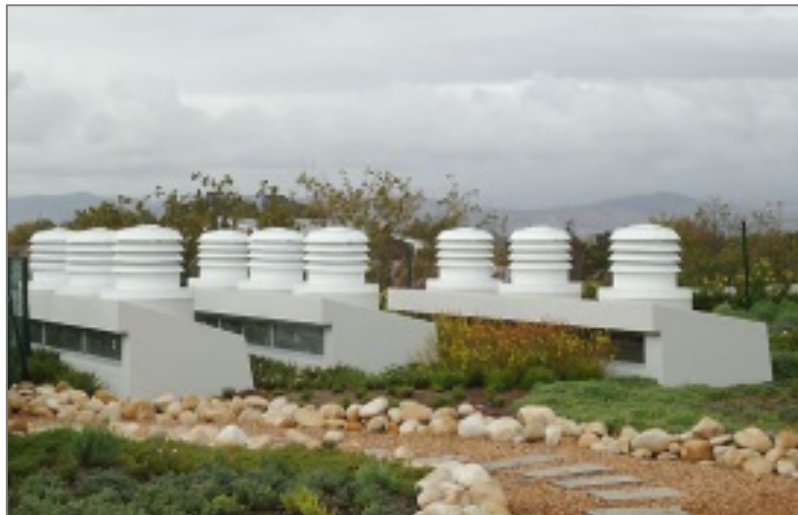
Figure 12 Prefab airtract ventilator utilizing venturi effect. 8
