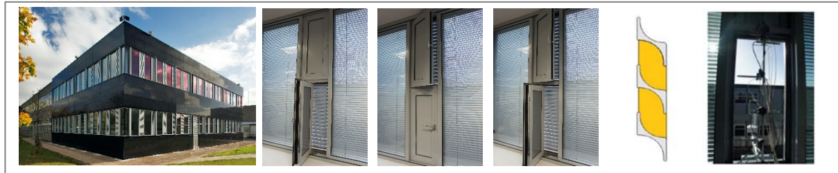
Figure 40 Building and ventilation system configurations. Left: configuration RS.02, middle: RS.03, right: RS.04. Configurations L1, L2, P1 to P3 in the middle are variations of RS.02.
