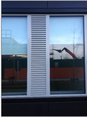
Figure 7 Examples of custom-made or project specific louvre solution. 3
