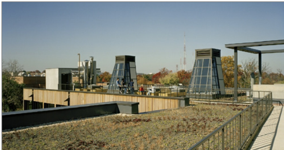
Figure 19 Solar ventilation chimneys. 15
