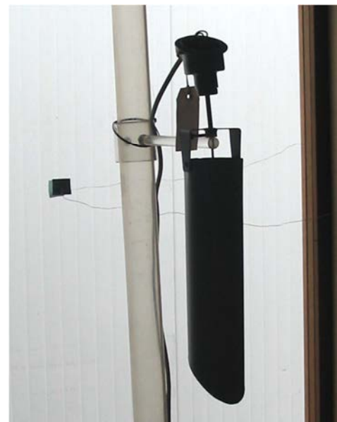
Figure 96: Air temperature measurement.
