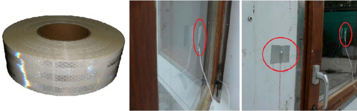
Figure 61: Detail of the recovering of the temperature sensors
