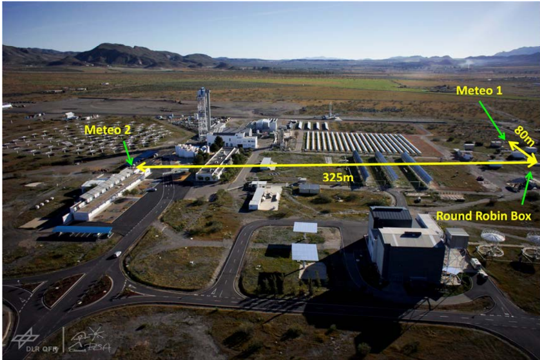
Figure 36: Location of the test box and the other meteorological devices at Plataforma Solar de Almería (PSA).
