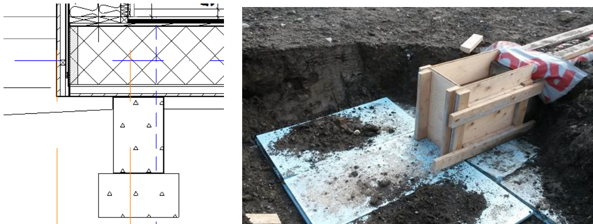
Figure 20. Details for the NO4 concrete foundation. The sketch is from the design stage (courtesy of Bergersen Arkitekter AS), and the photograph (courtesy of Marianne Rose Inman) is from the construction/as-built stage. Note the missing concrete pier foundation and additional insulation.
