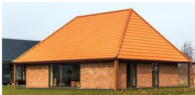
Figure 22. Design for long service life – traditional style. by Leth & Gori Architects [ @Jesper Ray, Realdania By og Byg ]
