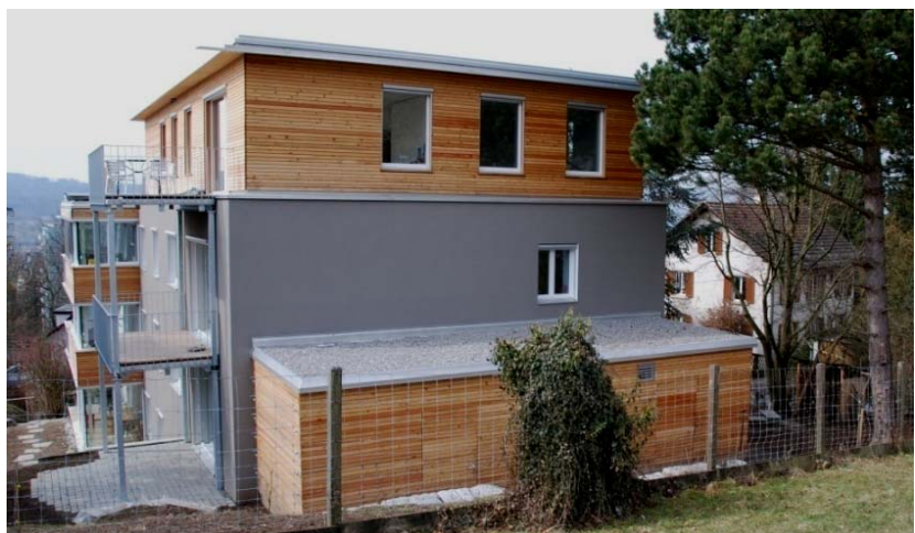
Figure 17: Renovated building from the north-eastern side. The building annex is used as technical space for the new heating system (ground coupled heat pump)
