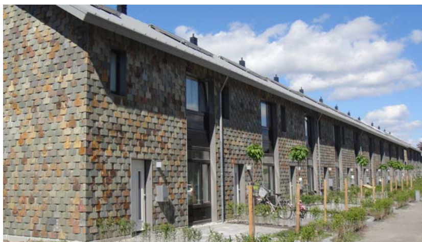
Figure 3: View of renovated building
