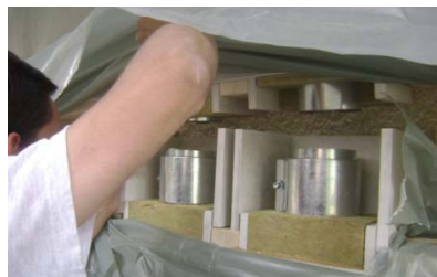
Figures 12-14: Ventilation main distribution with space saving rectangular ducts (top left), connecting the telescopic vertical round ducts between façade elements (bottom left), air inlet above window (right)
