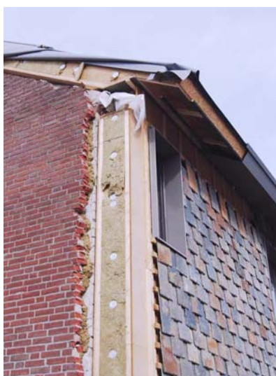
Figure 4: Section of renovated building
