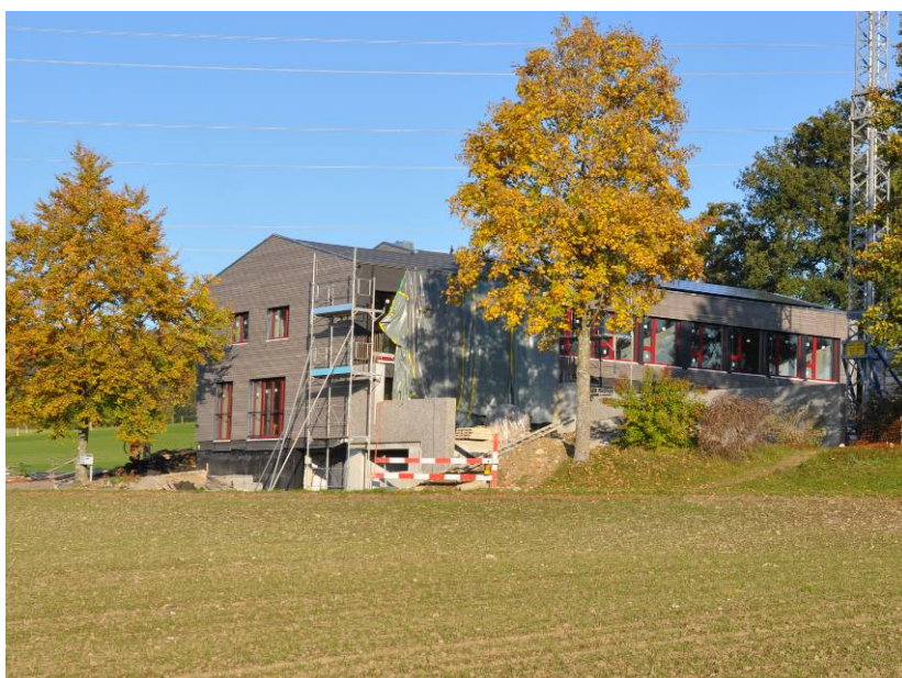
Figure 25: View of renovated building just before completion
