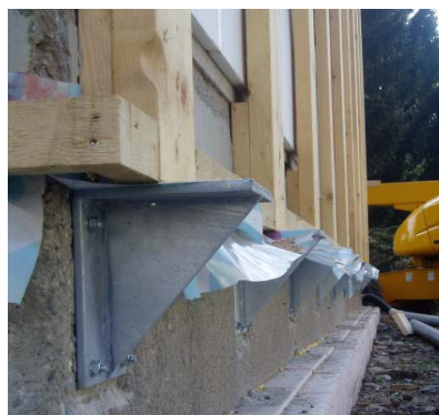
Figure 18: Steel-bearing angles on the plinth
