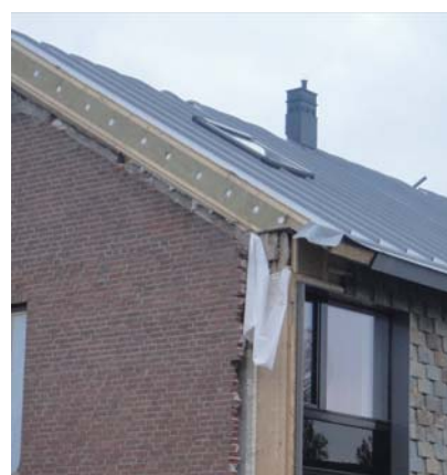
Figure 10: Prefab elements mounted on site
