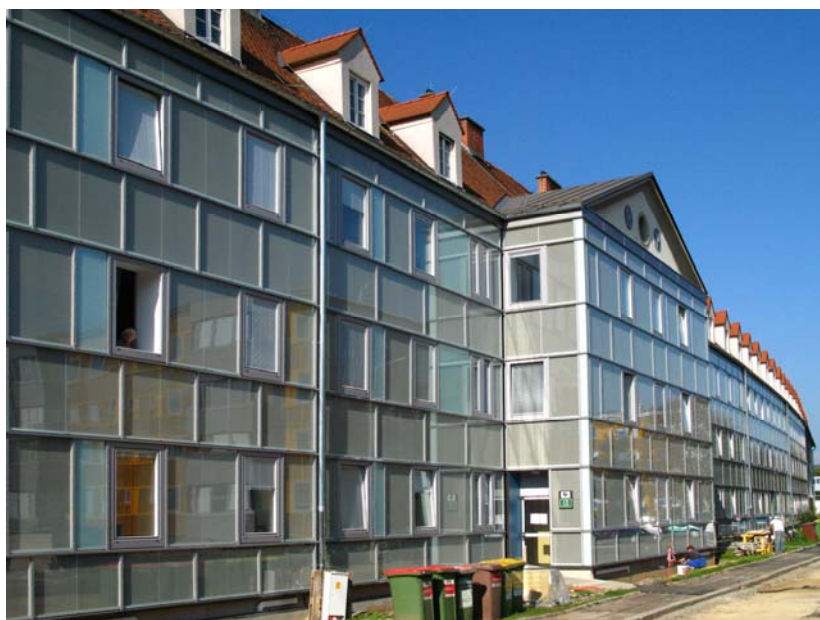
Figure 4: Dieselweg 3 and 19 – covered with new façade modules
