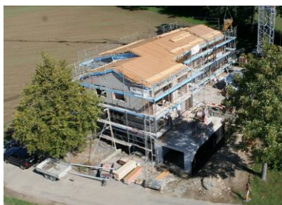
Figure 24: Areal view of the construction site, just before the façade elements were mounted (source: FHNW, René Kobler)
