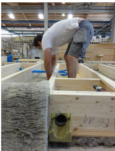
Figure 12: The timber frame construction is filled with sheep wool after the ventilation pipes and electric conduits have been mounted.
