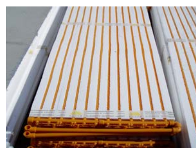
Figure 14: Heating pipes are inserted in XPS boards, which are mounted on the existing wall.
