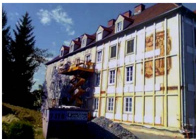
Figure 18: The on-site preparation is done by leveling laths. In-between the distribution system and supply pipes are installed.
