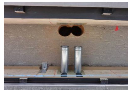
Figure 19-20: Horizontal mounting angle and a modules just before its final position
