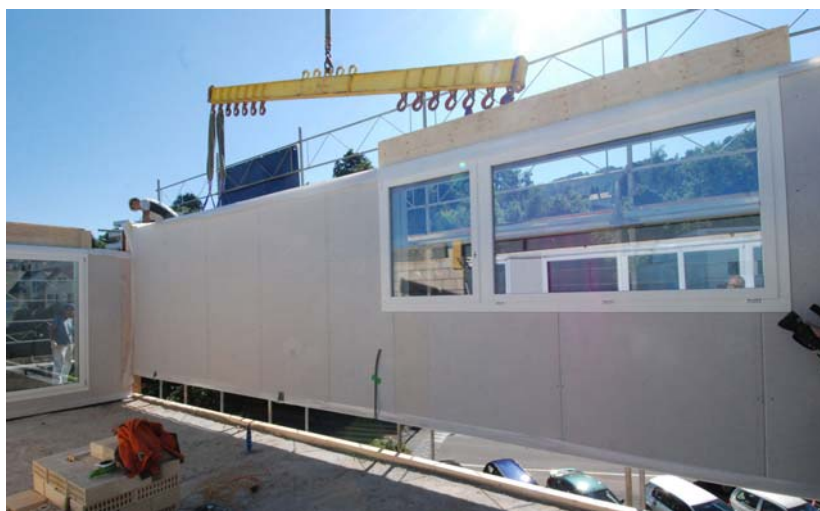
Figure 8: Mounting of the prefab structure
