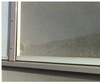
Figure 9: Solar comb protected by a toughened glass panel
