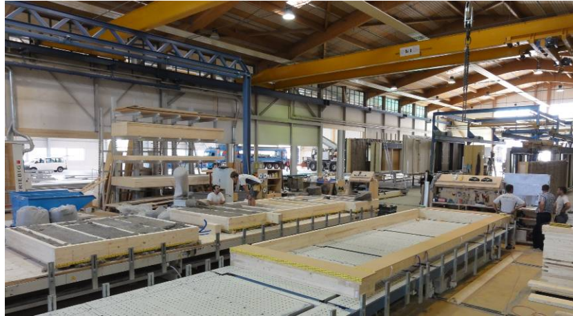
Figure 16: Prefabrication of modules in factory
