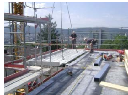
Figure 24: Mounting of the living room extension
