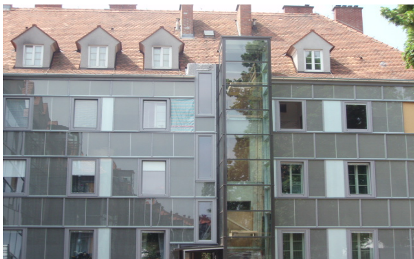
Figure 24: View of the renovated building from the back showing the additionally installed passenger lift
