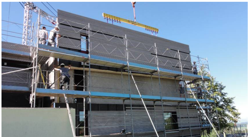
Figure 21: Mounting of the second module row
