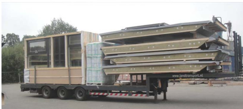
Figure 9: Prefab elements of one house at the factory
