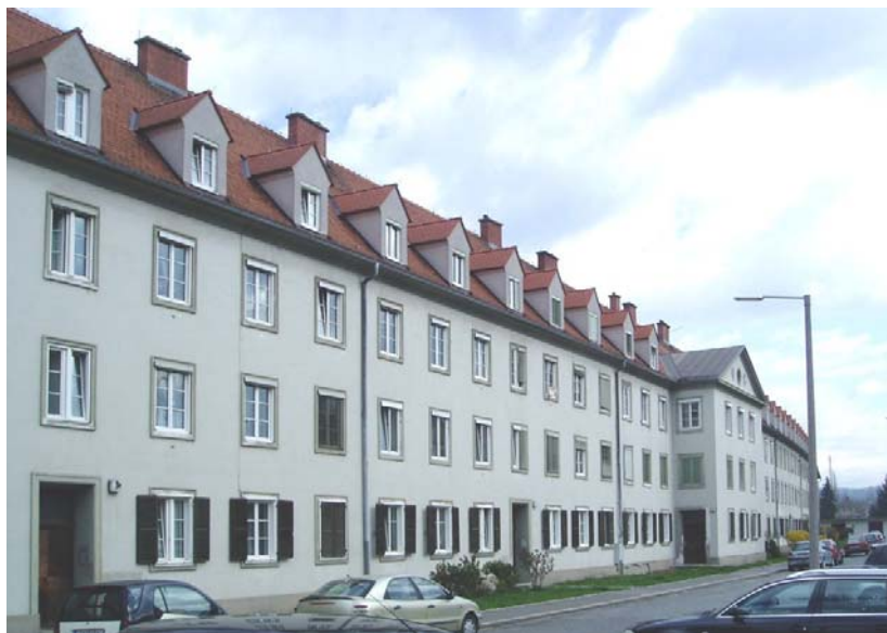
Figure 1: View of "Dieselweg 3-19" before renovation
