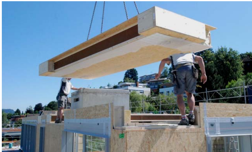
Figure 13: Mounting of prefabricated roof elements for new attic apartment
