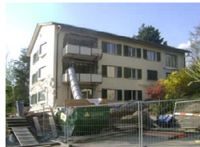
Figure 31: Apartment building just at beginning of renovation works
