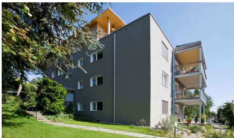
Figure 28: Renovated building from west side
