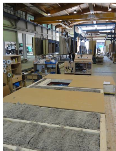
Figure 13: The insulated timber frame construction is closed with a medium dense fibre board.
