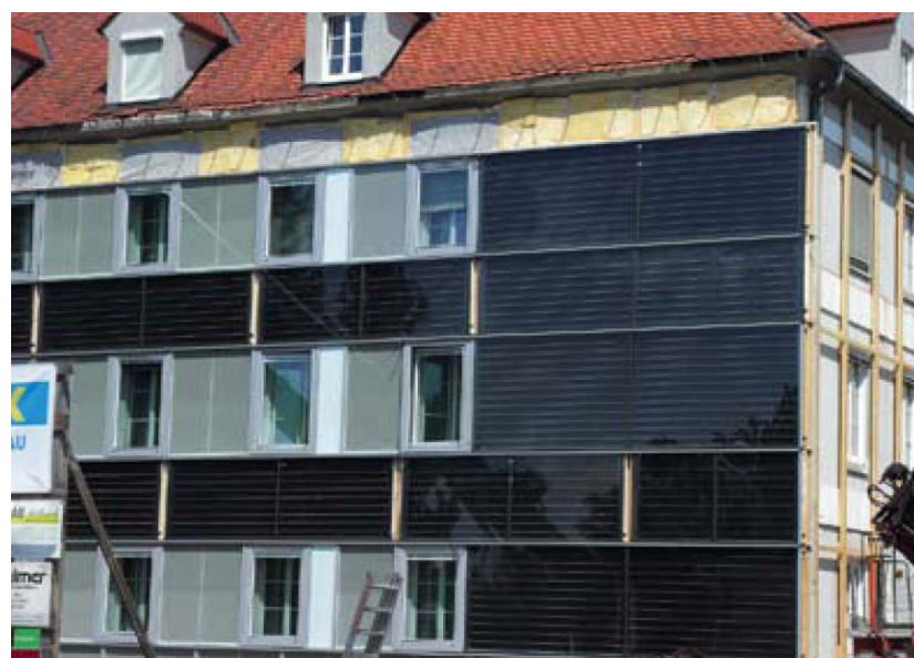
Figures 20-22: Sequence of assembly of the modules on the south-oriented façade (Source: Gap-Solution GmbH)
