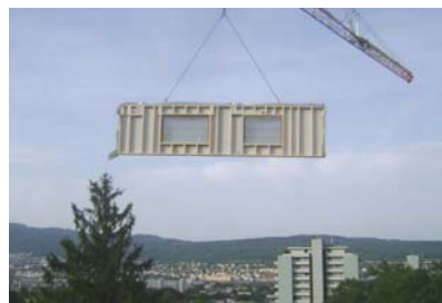
Figure 20: Mounting of 3 m by 10 m façade elements
