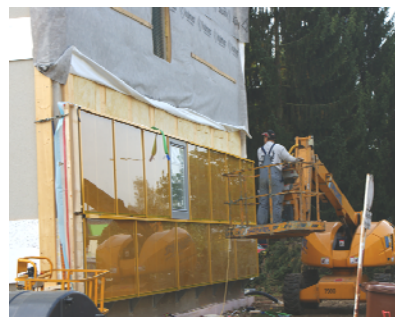
Figure 19: Assembly of lowest module
