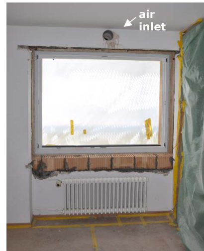
Figures 12-14: Ventilation main distribution with space saving rectangular ducts (top left), connecting the telescopic vertical round ducts between façade elements (bottom left), air inlet above window (right)
