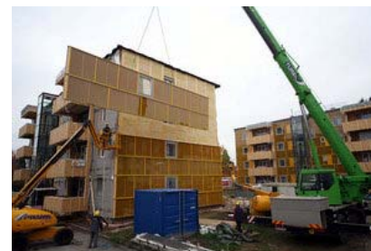
Figure 20: Mounting of 3 rd module
