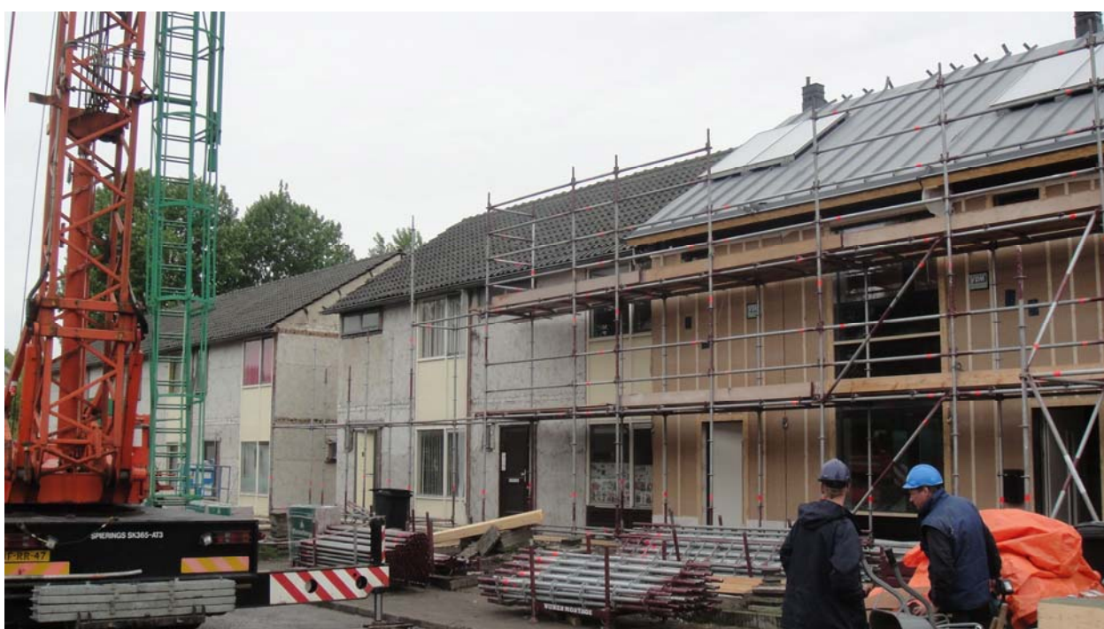
Figure 11: Renovation in progress: one house per day
