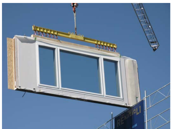
Figure 1: Prefabricated façade modules are used to construct a new building envelope around the building. This is physically optimal and does not reduce available space.
