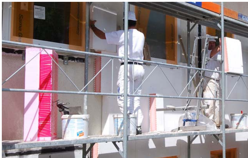
Figure 7: Insulation of façades with Hi-Compact insulation
