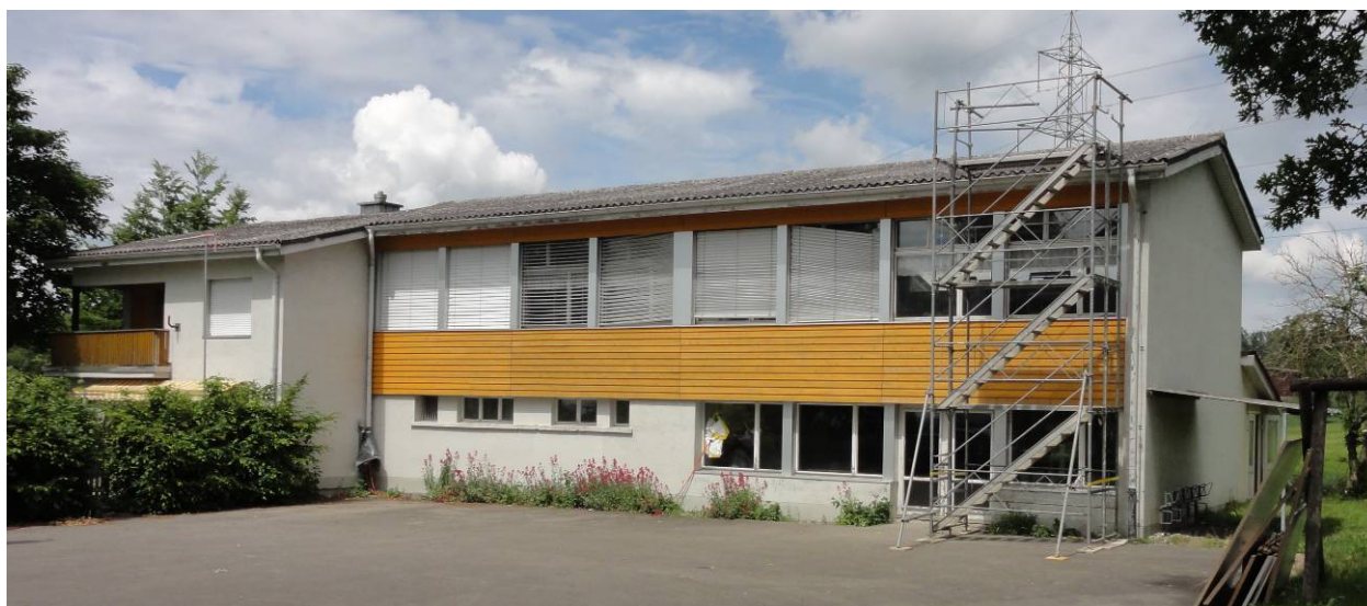
Figure 3: South view of the school building before renovation with the caretakers apartment on the left
