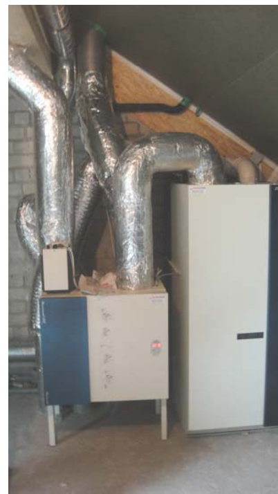
Figure 7: Combined heating, ventilation and hot water system
