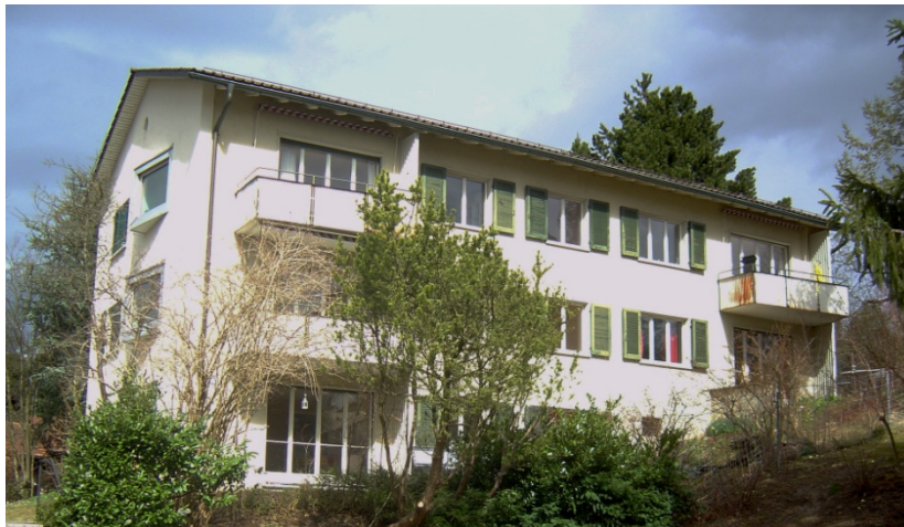
Figure 1: View of former south-east façade
