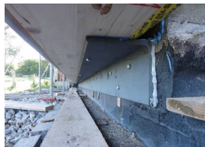
Figure 19-20: Horizontal mounting angle and a modules just before its final position
