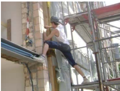
Figure 22: Preparation work for the living room extension
