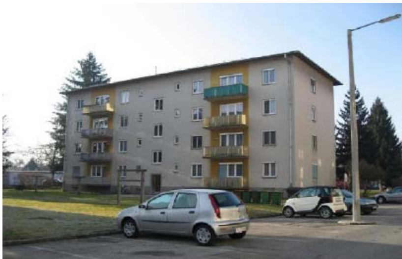
Figure 1: View of building (source: GIWOG)
