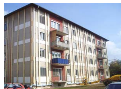
Figure 13: Heat distribution and XPS-boards are installed on existing façade
