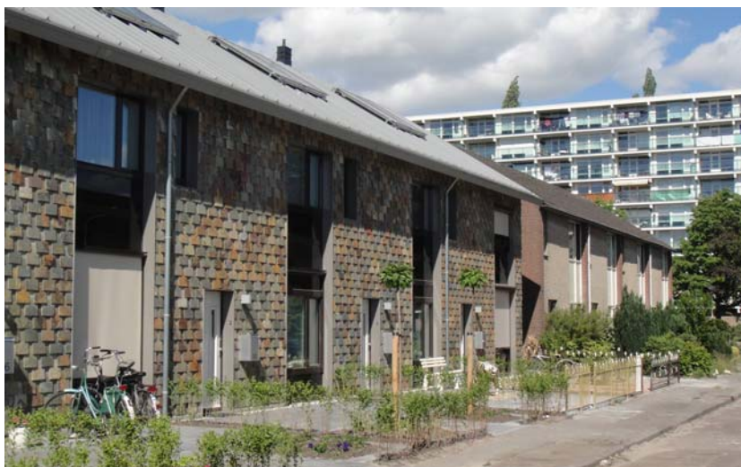
Figure 13: Impression of renovated and unrenovated houses
