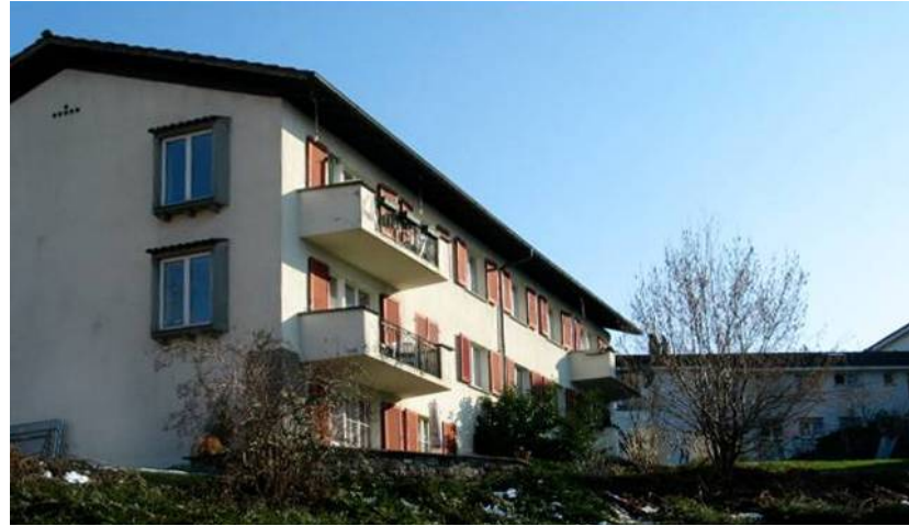
Figure 1: South-west view of apartment building before renovation
