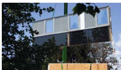
Figure 19: The solar collectors were integrated into the prefabricated modules. (Source: Gap-Solution GmbH)
