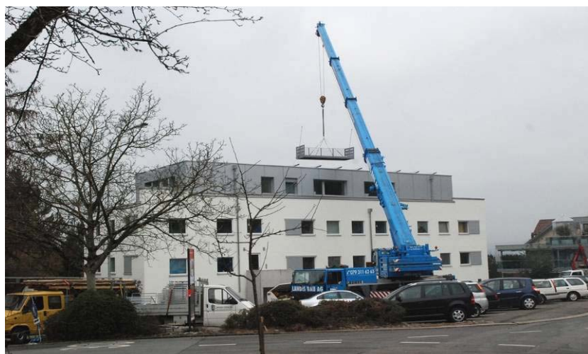
Figure 15: Mounting of pre-fabricated balconies
