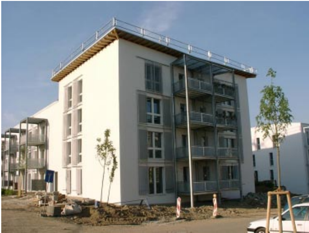
Figure 2: A CEPHEUS project in Kassel, Germany: Two multi-storey apartment buildings totalling 40 units were built here by GWG Kassel on the site of a former military barracks. Three teams of architects (Prof. Schneider; HHS; ASP) designed the buildings. Vacuum insulation panels are used in some casement doors as opaque filler panels.
