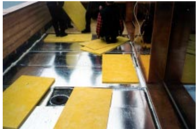
Abb. 3b: Completion of the terrace using 5 cm thick vacuum insulation panels
