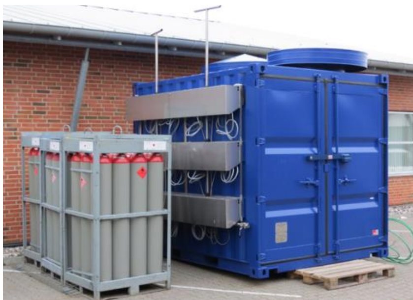
Figure 68. A 50 kW LT-PEMFC CHP hydrogen unit from Dantherm Power [3].
