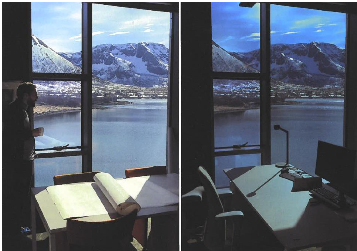
Figure 52. Left: When there is no need for solar shading, the glasses are light and transparent like ordinary windows. Right: When there is a need for solar shading, electricity is applied to the nanocrystalline film and the glass turns darker [2].
