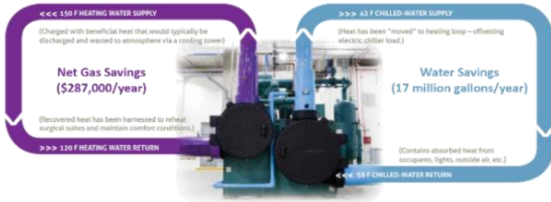
Figure 143. The heat pump chiller saves $287,000 per year in gas savings and 17 million gallons per year in water savings. 6
