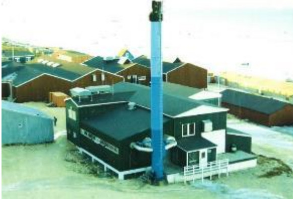
Figure 69. Cooling fans on the roof are now used only for emergency (Source: Nukissiorfiit).
