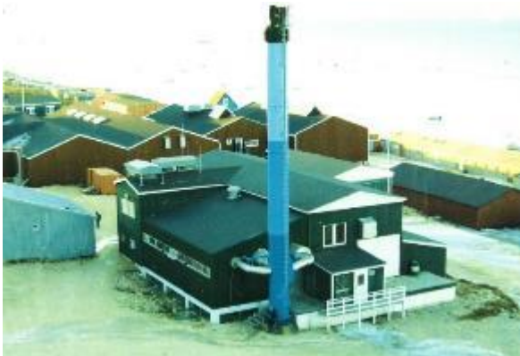
Figure 69. Cooling fans on the roof are now used only for emergency (Source: Nukissiorfiit).
