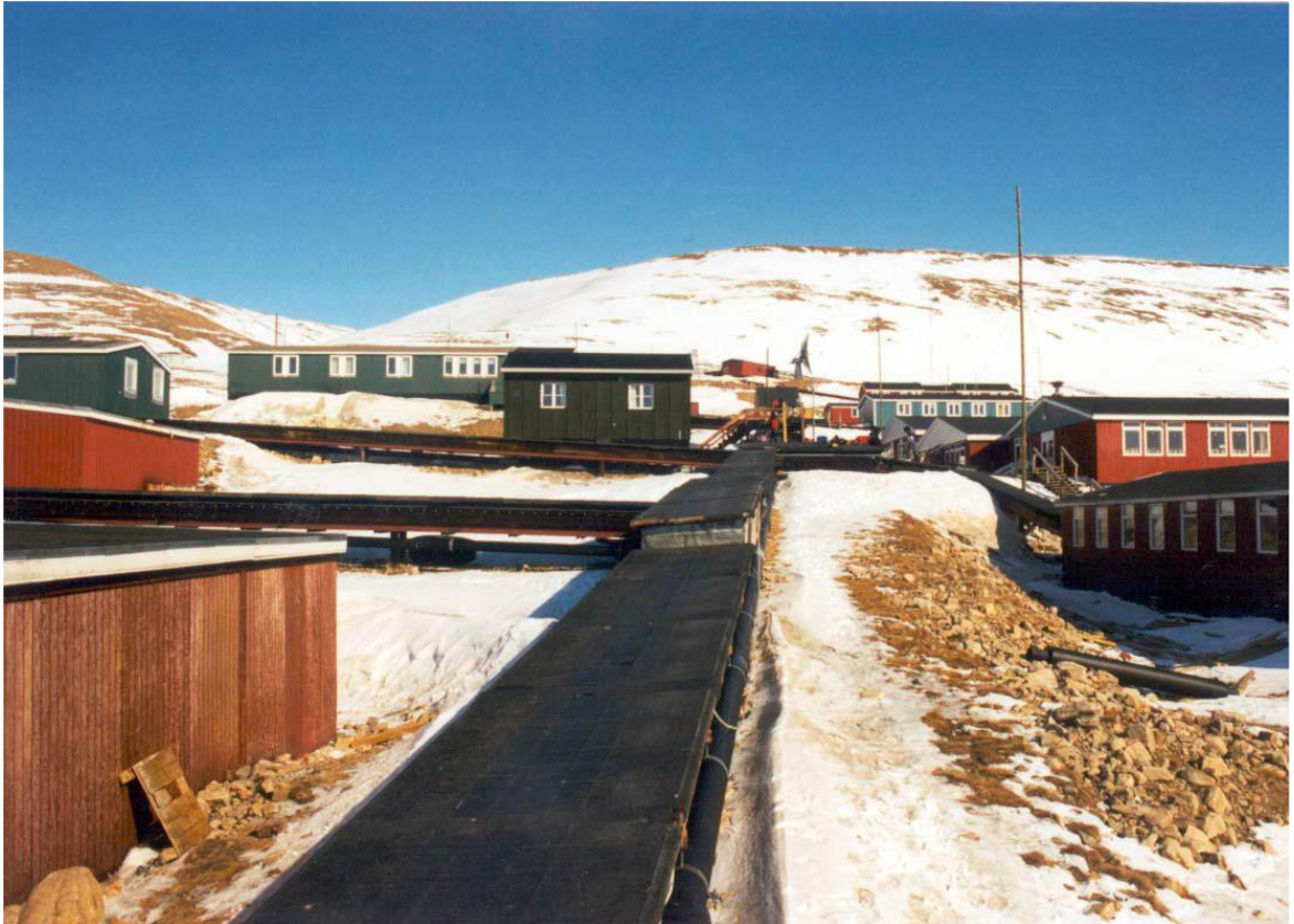
Figure 70. The infrastructure in Quanaap, Greenland, is above ground due to permafrost (Source: Nukissiorfiit).
