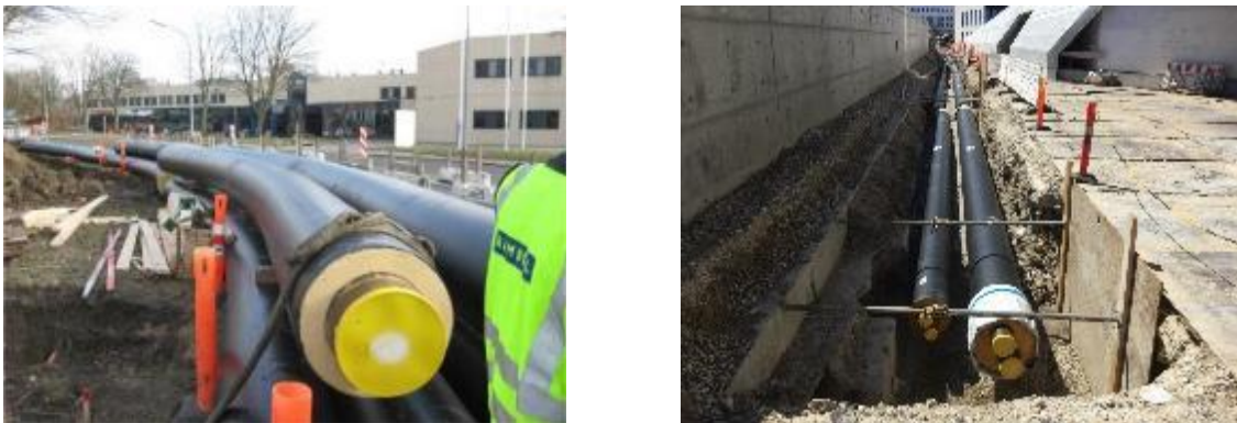
Figure 45. District heating pipe construction, with curved pipes(left) and straight pipes (right) (Source: Ramboll).
