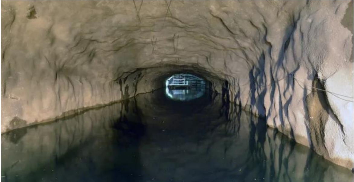
Figure 106. Underground water cooling reservoir in Esplanade Park located at a depth of 100m (Photo by Pekka Nieminen from Helen cited in an article by Walker, https://gizmodo.com/helsinki-built-an-underground-lake-to-cool-its-building-1631985837 ).
