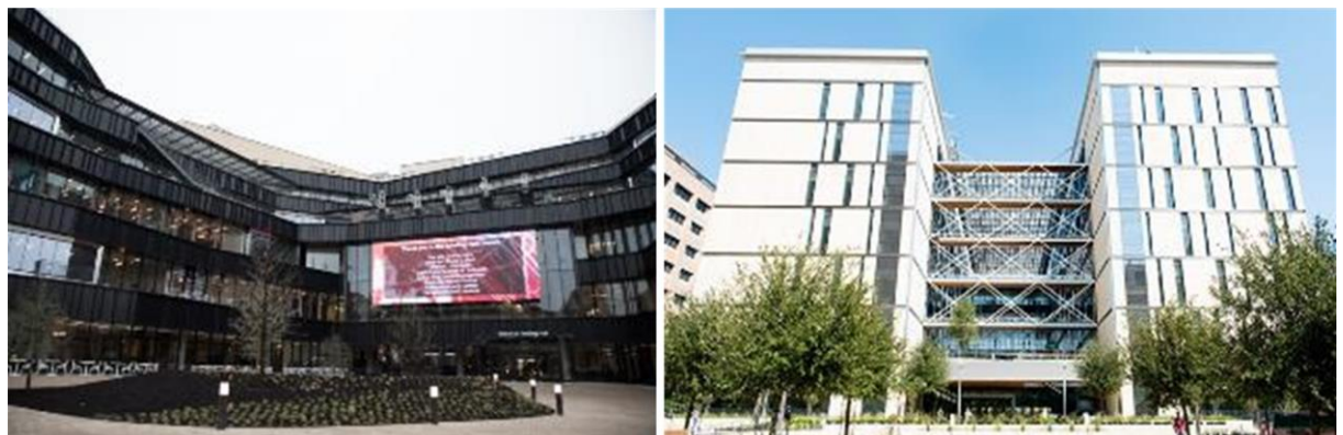
Figure 141. Chilled water and heating connections for the Graduate School of Business and the Engineering, Education and Research Buildings at the University of Texas Austin. This connection is via direct connection to the Main Campus looped chilled-water and steam tunnel distribution system.
