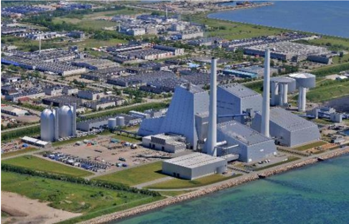
Figure 49. The Avedøre multi-fuel CHP plant with heat storage tanks (Source: Ramboll).
