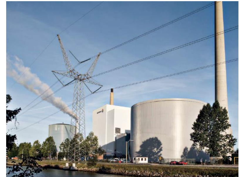
4TH GENERATION DISTRICT ENERGY 06-12-2017
