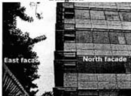
Energy Efficient Buildings in Tropical Climate IEA Futures Building Forum Oslo 09 - 11 May 2001
